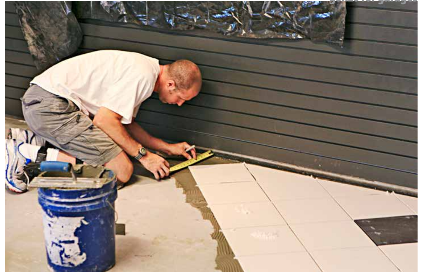
Chad chose porcelain tile for his floor. The installer centered and marked the design in the middle of the floor so that the partial tiles abutting the most visible wall would be triangles of the tiles cut in half diagonally, creating the diamond pattern Chad wanted.
