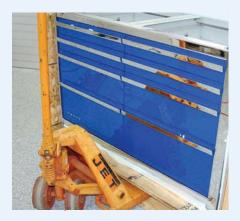
7. With cabinet in positon and using a level, raise and lower leg levelers until it is level with the floor and adjoining cabinets.
