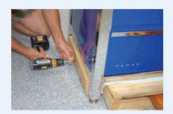
5. Using a pallet jack, raise cabinet and screw leg levelers into the bottom of each frame.
