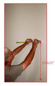
4. From that mark, extend a level layout line along the wall by snapping a chalk line, using a laser level or marking along the straight edge of a carpenter's level. Here again, if the floor is sloped you may need to make adjustments. This layout line will establish the height on the wall where the upper mounting bracket will be installed.
