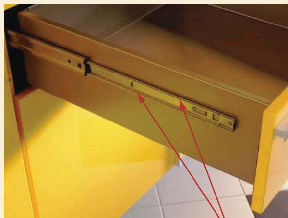
This is the drawer slide "travel" and location to place a small amount of white lithium grease.
